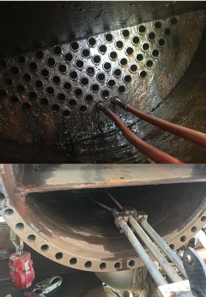
Fouling components and rust gradually form during operational processes that will eventually require removal. Our high-pressure washing equipment is designed for various industrial applications that will leave equipment surfaces free of deposits and rust.
