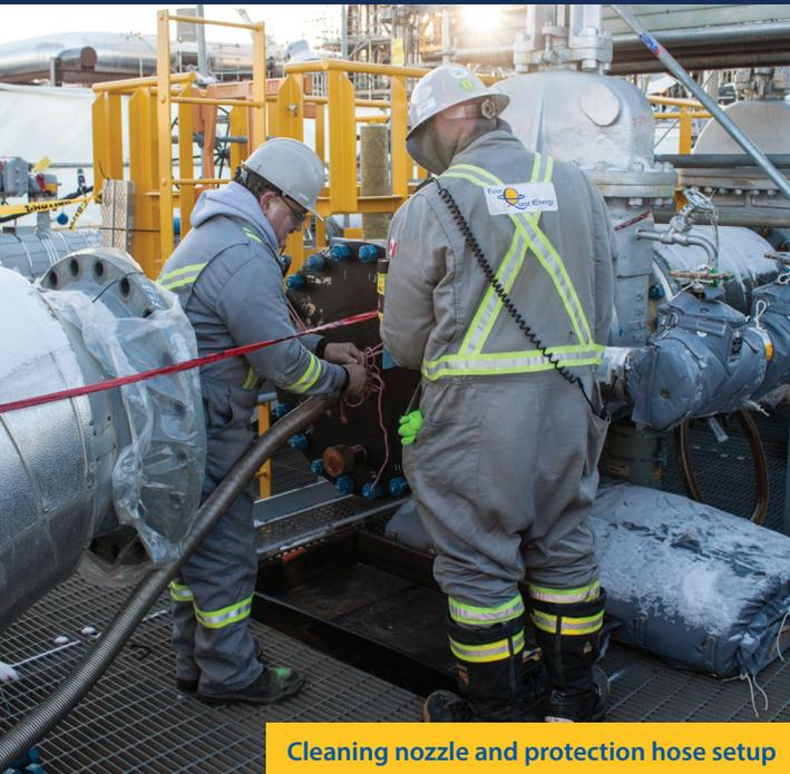
Cleaning nozzle and protection hose setup
